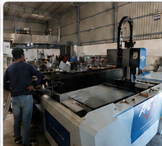
FABRICATION WORK IN PROGRESS
