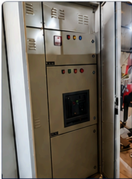
ELECTRICAL PANEL FABRICATION
